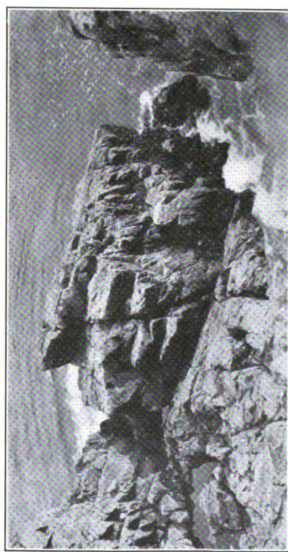
JOINT CONTROL OF SEA EROSION. FIGURE 8.
